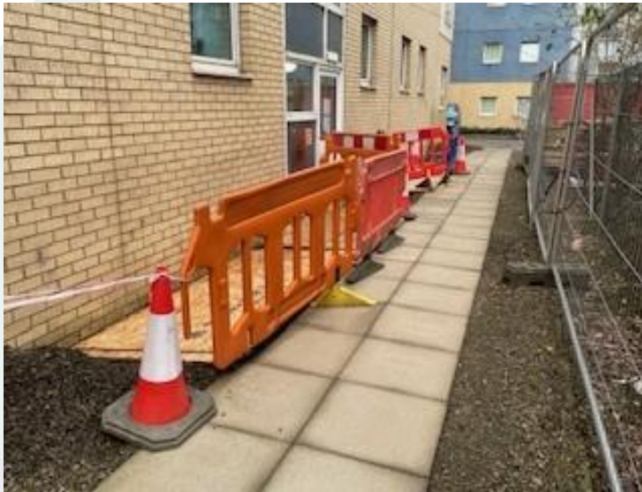
Blockwork foundation phase 4
